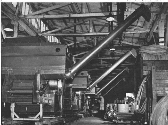
The production line for making pre-cast concrete panels which are used in many Housing Commission building projects.
